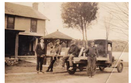
Part of the work crew
