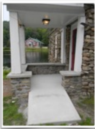
Masonry work completed
